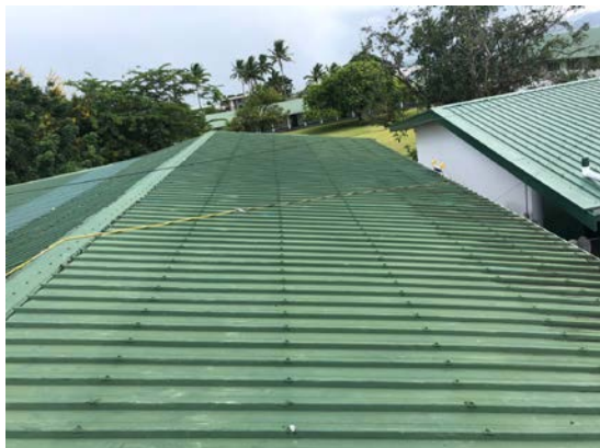
(Above: Old roof)
