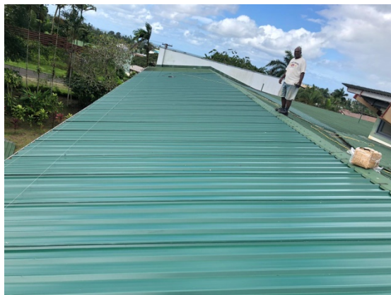
Above: New roof and contractor admiring his work
